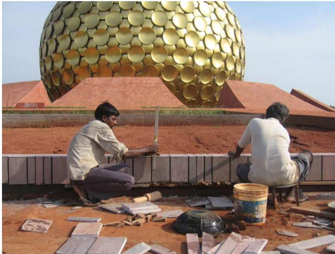
The work of cladding the low walls in the garden of Bliss with slate stone slabs begins
