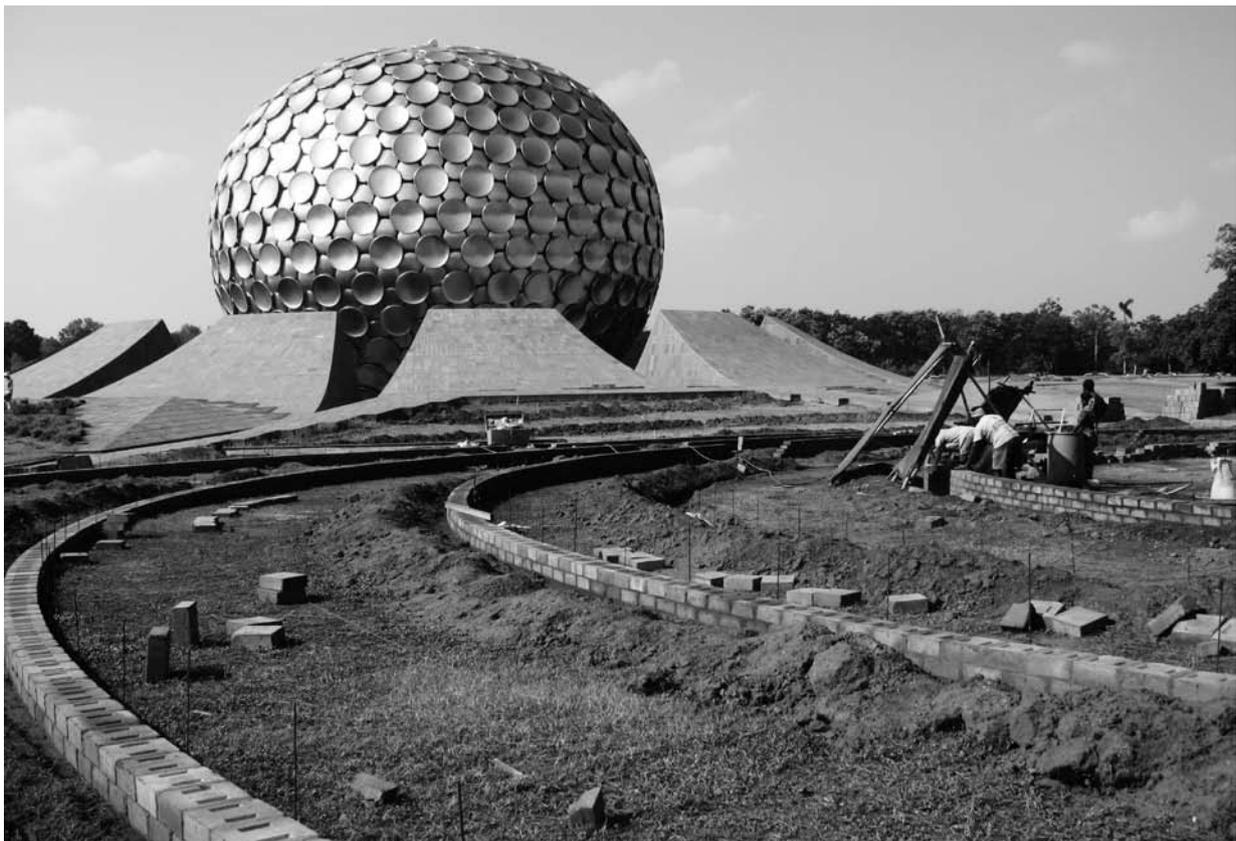
Building the compressed earth block walls in the garden of Bliss
