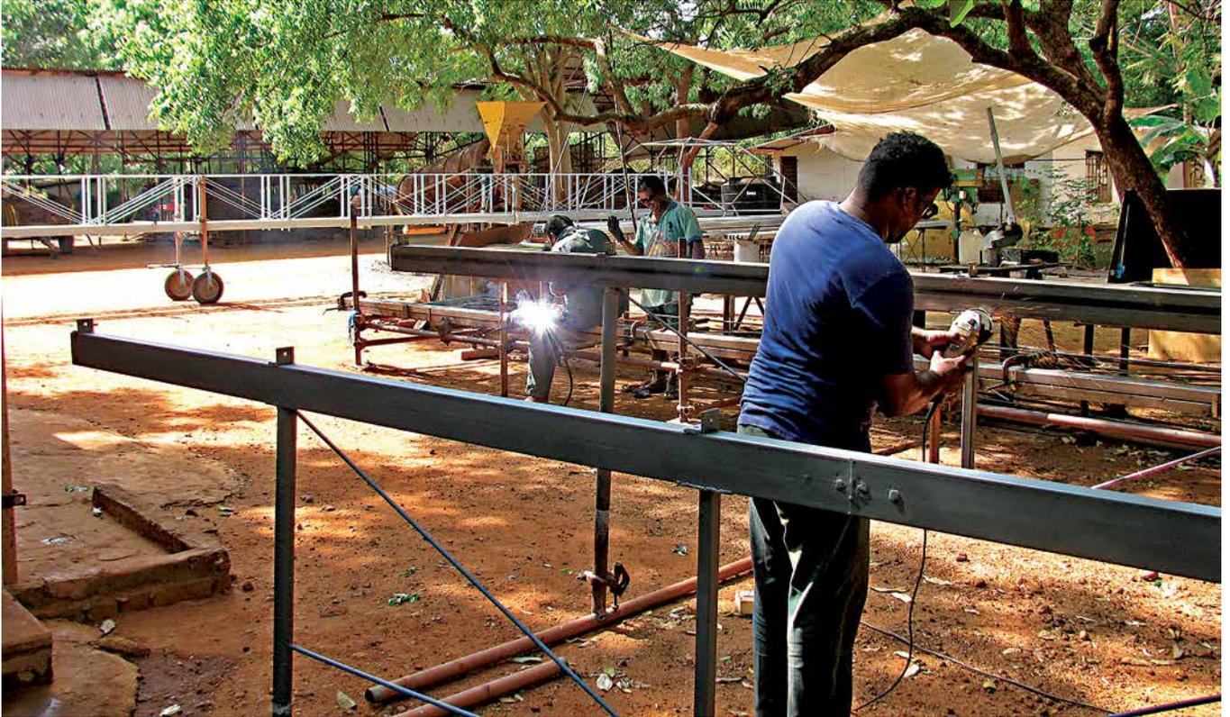
*Roof trusses for the new compost shed are being manufactured in the Matrimandir metal workshop.*
