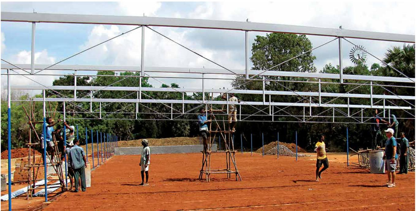
*The Matrimandir metal workshop team installs roof trusses for the vermi compost production shed at the new site.*
