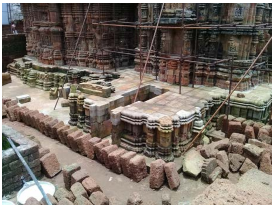
Examples of laterite block (above), and laterite block uncovered during an archaeological excavation at Vabanishankar Temple in Bhubaneswar (below)
