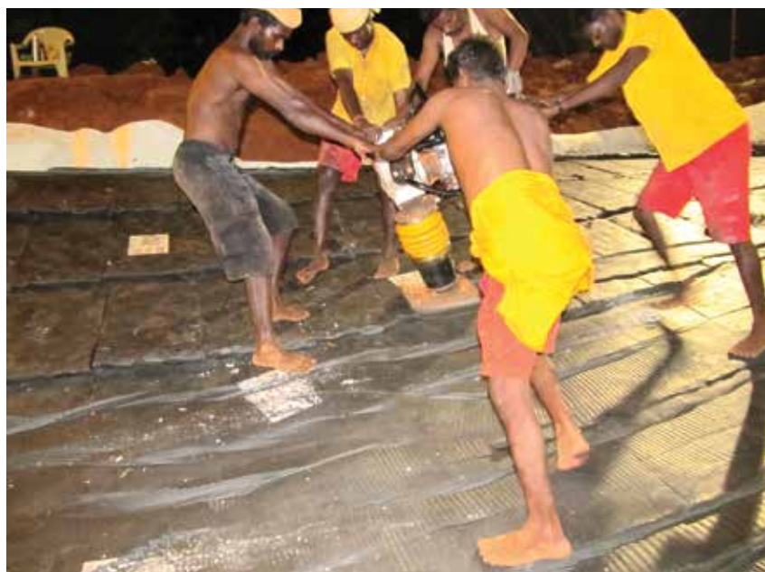
A "pogo stick" jumper is used to knead the clay slabs so they join and become one waterproof layer.
