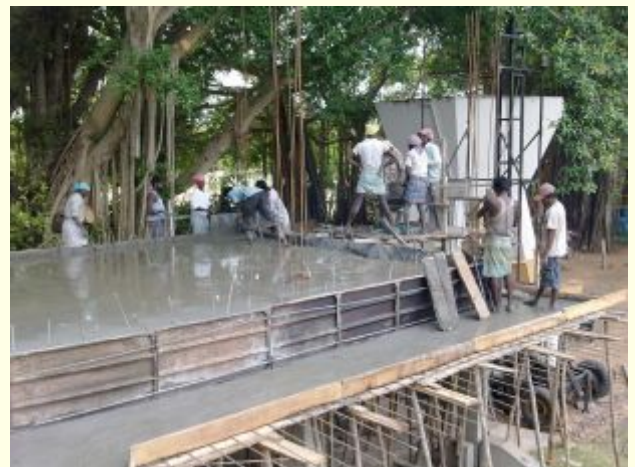
The concrete was poured in 1 day
