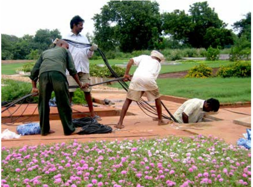
Electric cables powering pumps and lights in the first three gardens are rerouted under the pathways to go to the new underground control room in the Garden of Consciousness.
